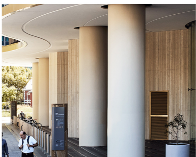
05. Columns Applied textured finish
