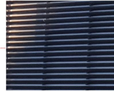
06. Plant Ventilation Charcoal grilled louvre system
