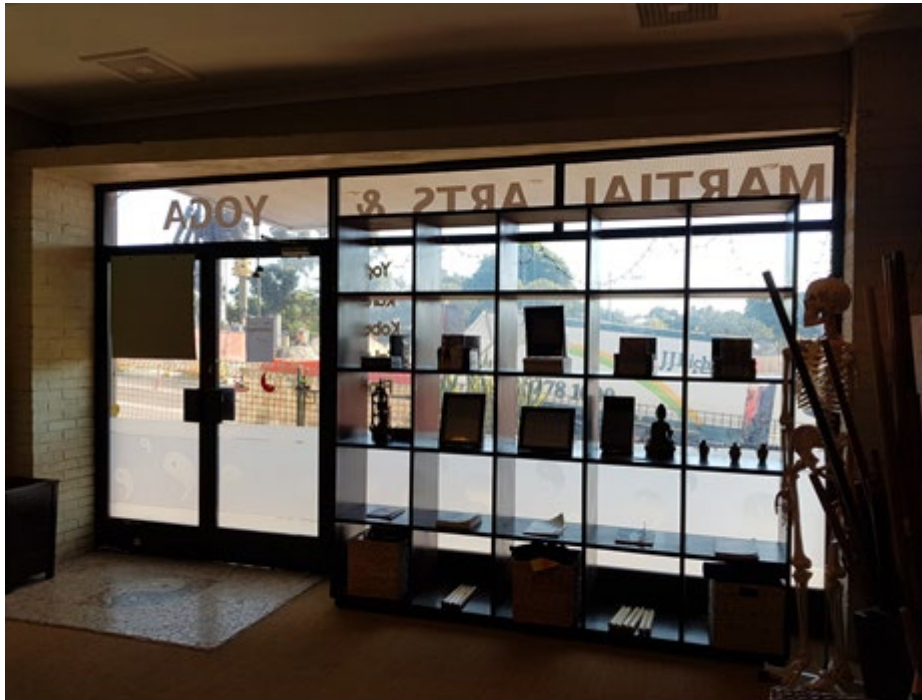
Figure 6 Existing Interior Shopfront
