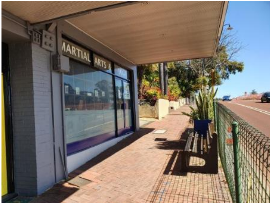
Figure 10 Existing Glass Front Signage
