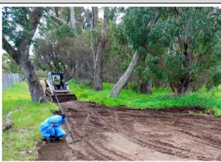
**Photograph 2:** Western access track ACM impact area - hand picking, raking, and excavation (facing north)
