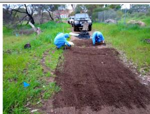
**Photograph 1:** Western access track ACM impact area - hand picking and raking (facing south)
