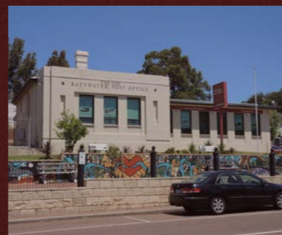
7. The Old Bayswater Post Office
