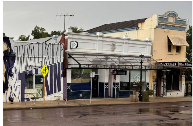
Figure 3 existing condition of neighbouring contributory heritage building no13 & 15 King William Street located east of the subject site.
