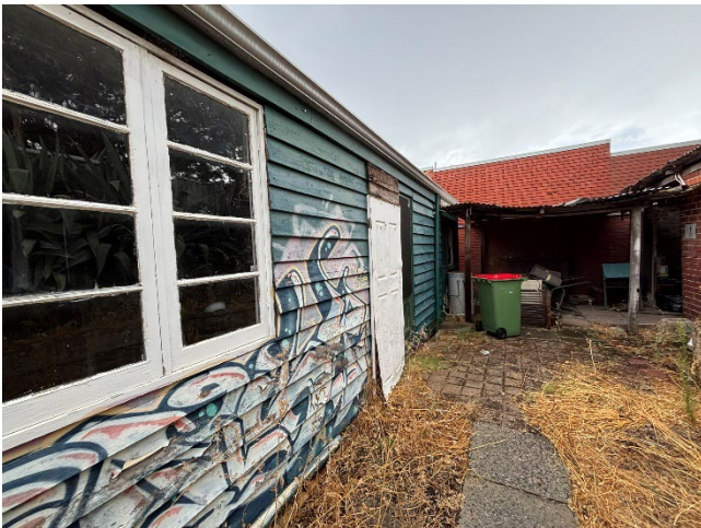
Figure 6 North (rear) elevation of 9 King William Street Source: Urbis 2026
