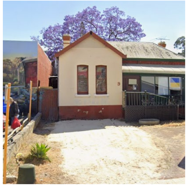
Figure 21 – Photo taken after removal of the finials, dated November 2023.
