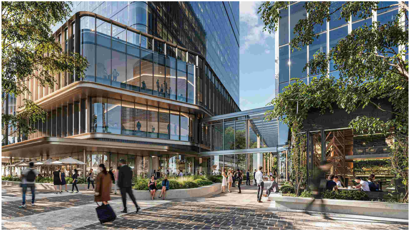
VIEW FROM GALLERA ENTRY (SOUTH)
