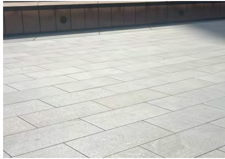
Pedestal paver on podium
