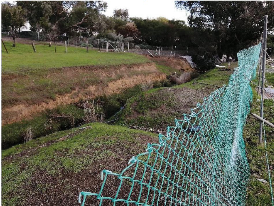
Photograph 6: View of existing Neerigen Brook along the southern boundary
