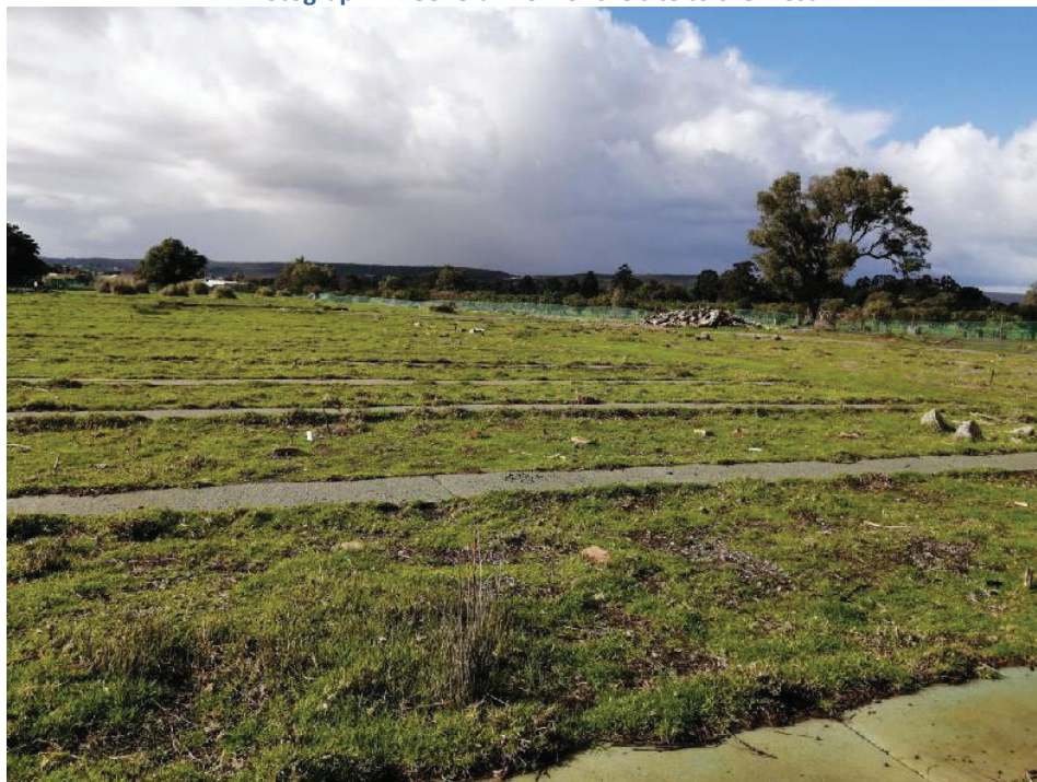
Photograph 2: Concrete slabs (possible strip footings) on the western side of the site
